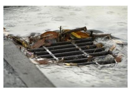
and natural conveyance in the form of infrastructure such as creeks, culverts, detention basins, drywells, pipes, localized treatment systems, and storm drain inlets. This infrastructure collects stormwater, and in some instances partially treats it, before the stormwater is discharged to either groundwater or surface water.
