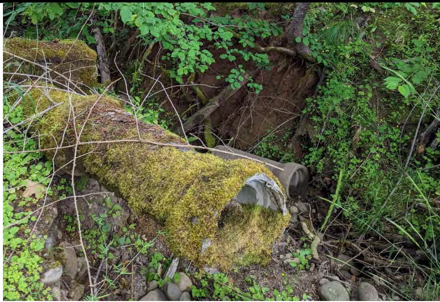
Photo point 16. Photo 1. Top of stormwater outfall gully, facing downslope at old culvert segments that have become disconnected due to undercutting of soil
