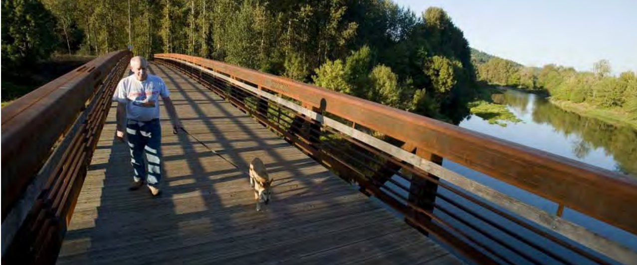
Washougal River Greenway Bridge, Camas, WA
